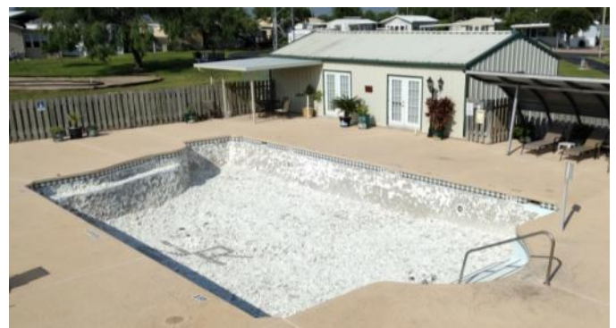
A Dry Pool with the Plaster Removed.
