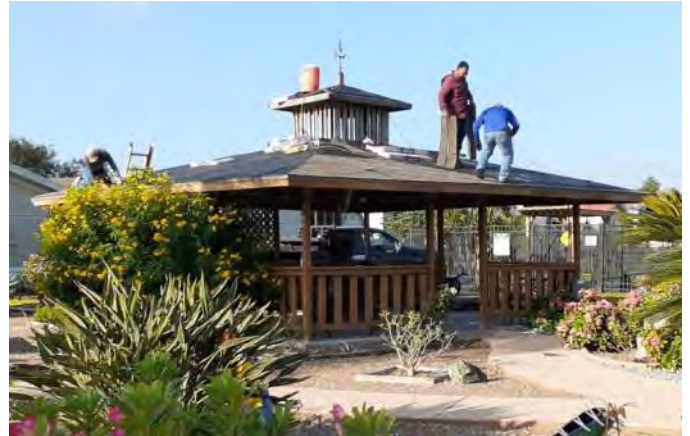
A New Roof for the Gazebo
