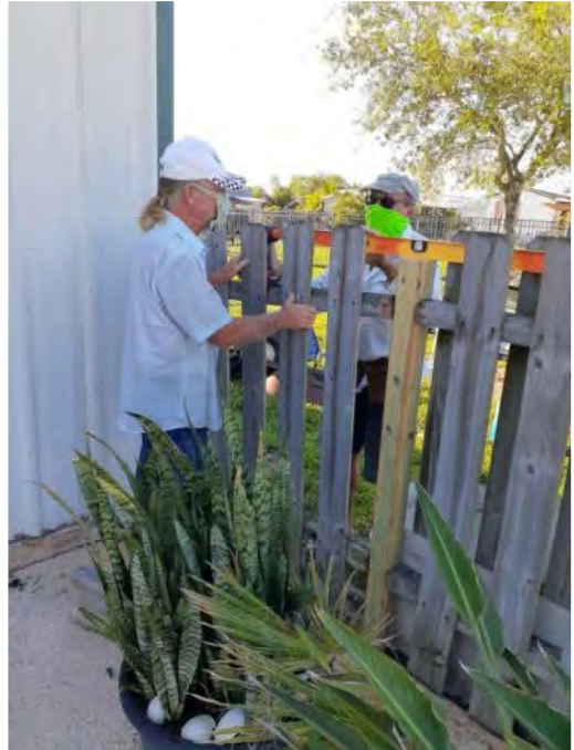
Repairing the Pool Fence
