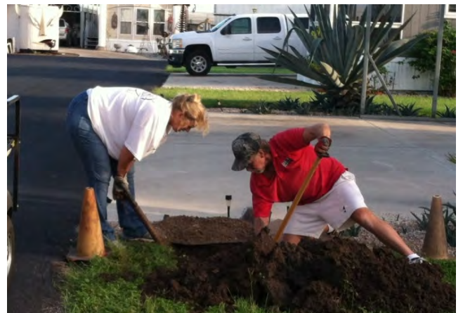
Excavating to Find the Leak.
