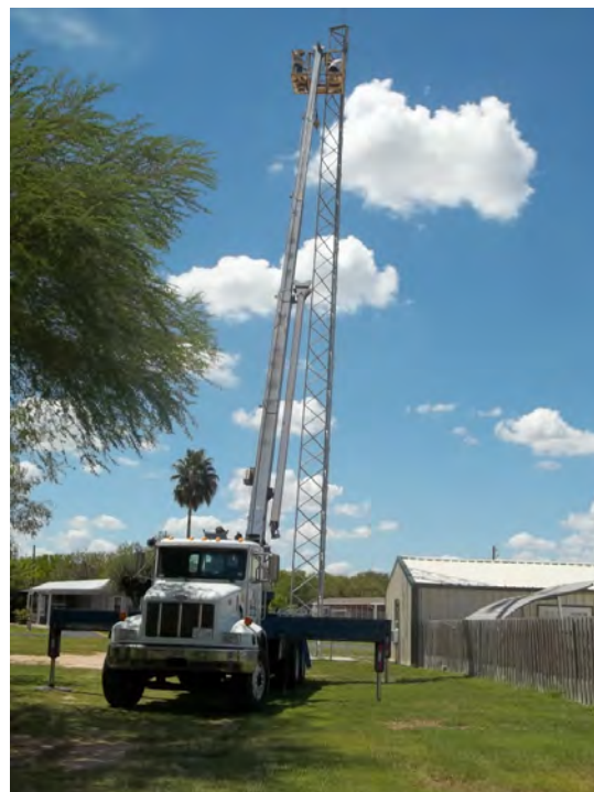
Putting up the Point to Point Receiver
