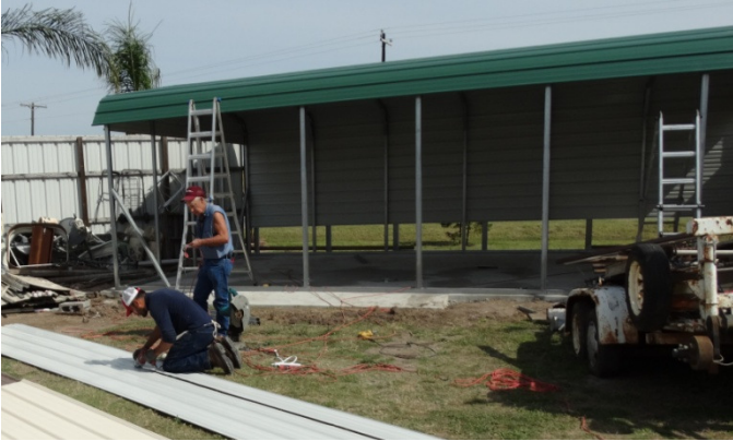
Putting up the Walls
