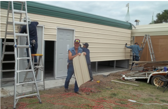
Framing and installing doors.
