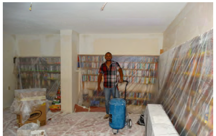
A New Ceiling in the Library
