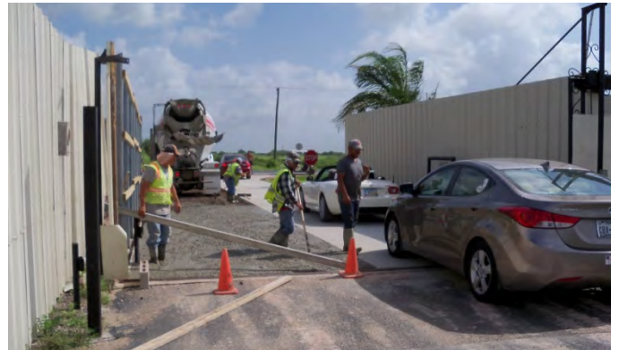
Navigating through Driveway Construction
