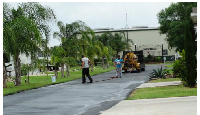
Sealing the Driveway
