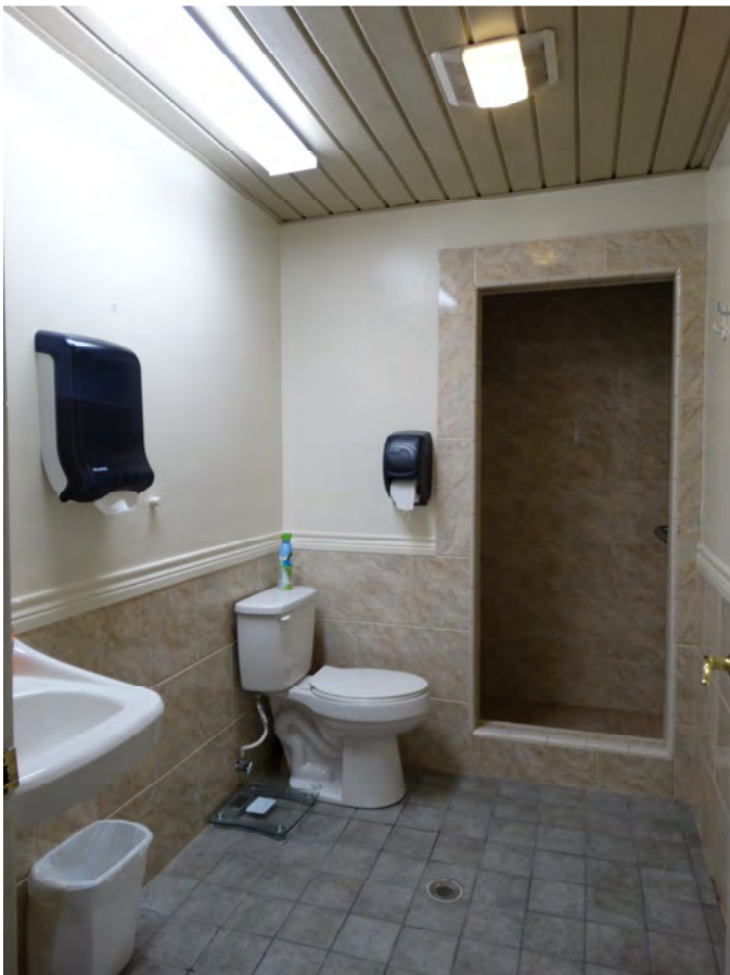
The Job is Complete and the Showers and Bathrooms look Great!
