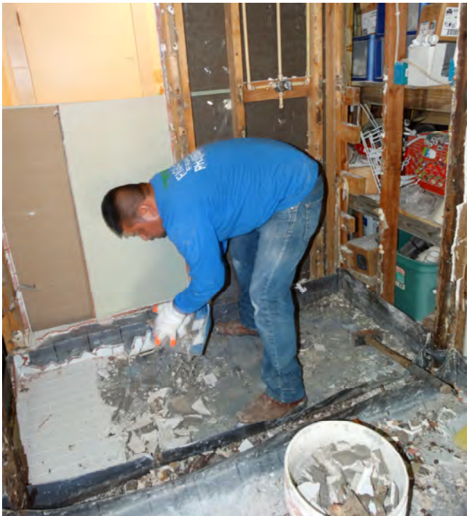
Tearing out the old showers including the cement floor
