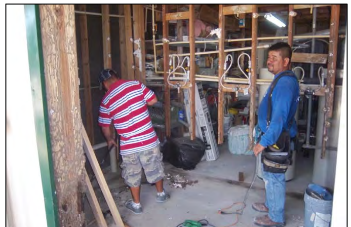
Tearing Down the Walls of the Outside Shower
