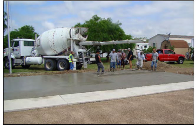
A New Pickle Ball Court being Poured!
