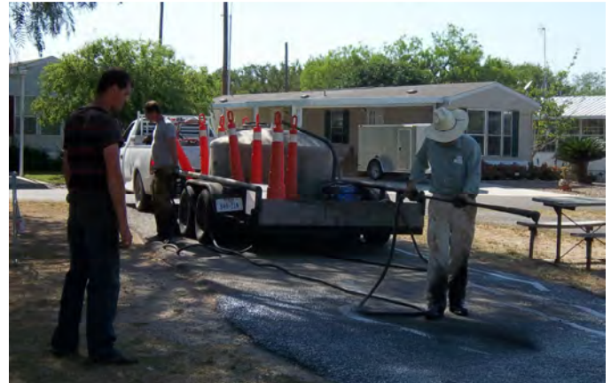
Seal Coating the Pull Throughs
