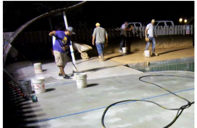
Pouring Cool Deck at 4 a.m.
