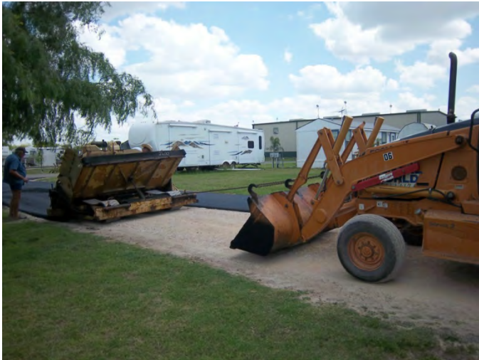
Note the Chain linking the Paver to the Backhoe!
