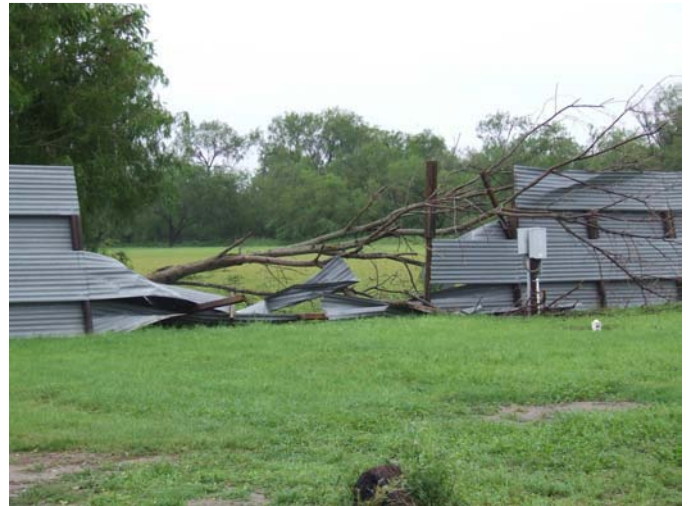
Damage by Hurricane Dolly
