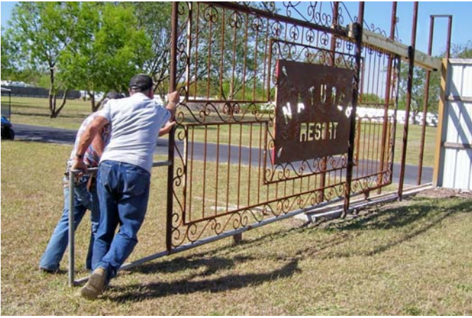
The New Gate goes in
