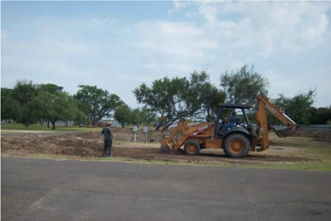
Installing a Septic System – Phase III
